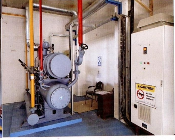
SRM Screw-type Ammonia Compressor
