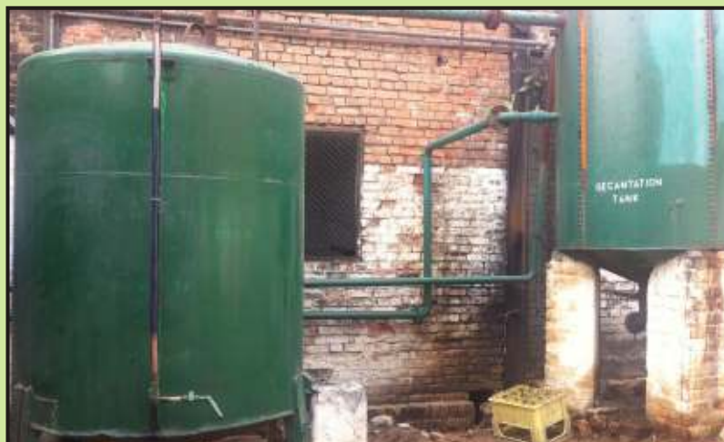
SLUDGE SETTLEMENT SYSTEM
