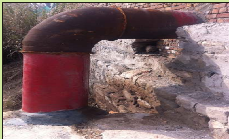
OUTLET DRAIN TO NALLAH LAHI
