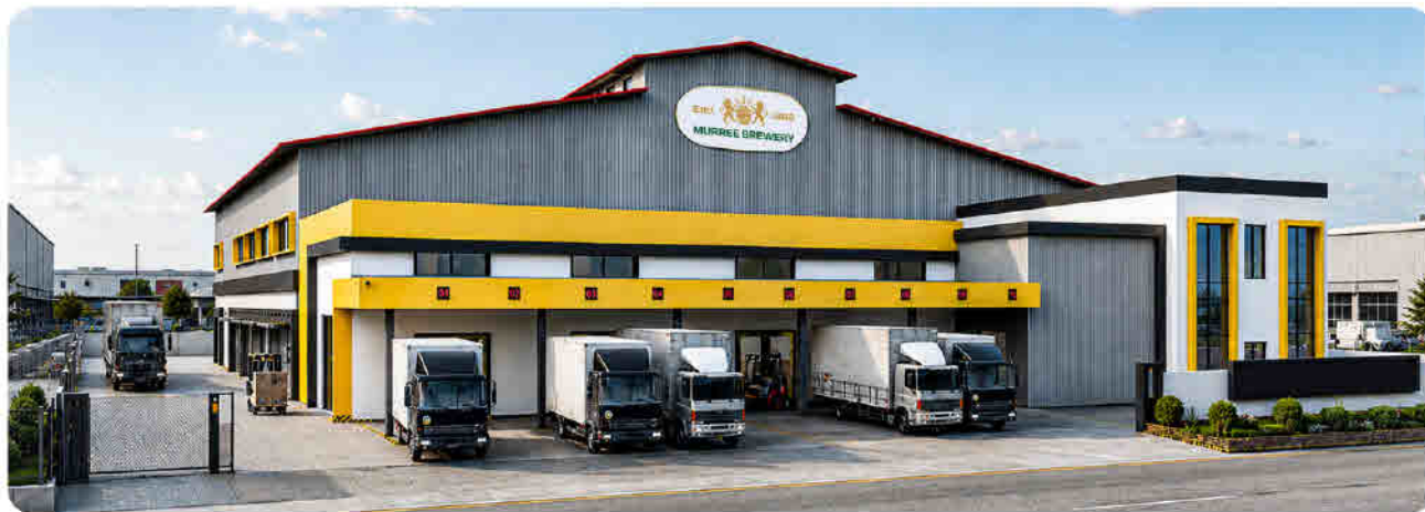
New Factory Site for Carbonated Soft Drinks in Hattar, KPK - Capacity Expansion in Progress
