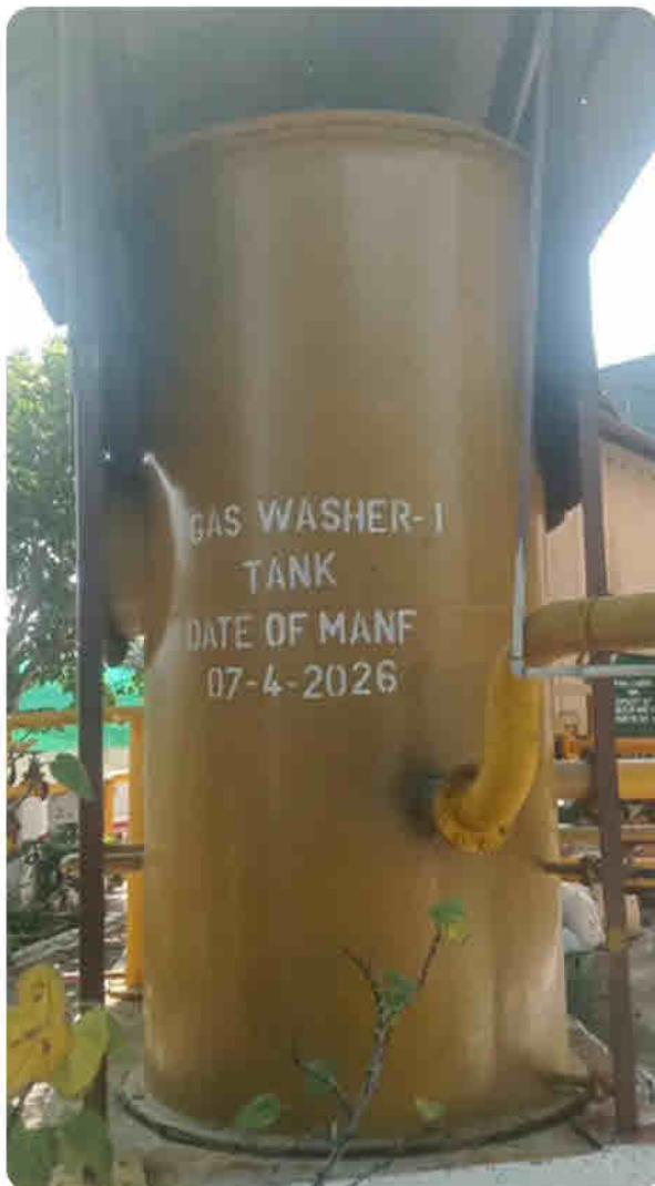
Wastewater Treatment Upgrade to Remove Sulphur Pollutants
